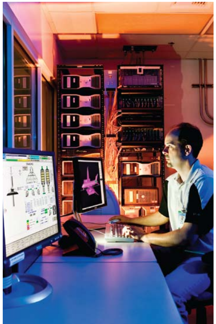
PHOTO: Neil Kuntz, automation designer for Everett Site Services Plant Engineering, monitors systems from the control room of the 45-03 widebody paint hangar at the company's Everett plant. The newly installed systems are linked to a computer network that is used to manage the hangar's operations. GAIL HANUSA/BOEING
